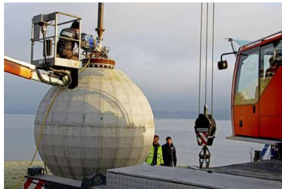
Fraunhofer's 3m concrete sphere Andrews (2018) A review of underwater compressed air storage
